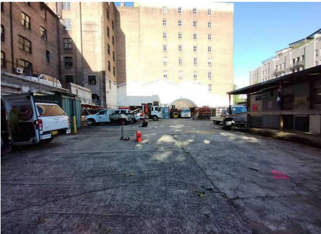
Photo 16: Concrete surface across the site - Looking south-west
